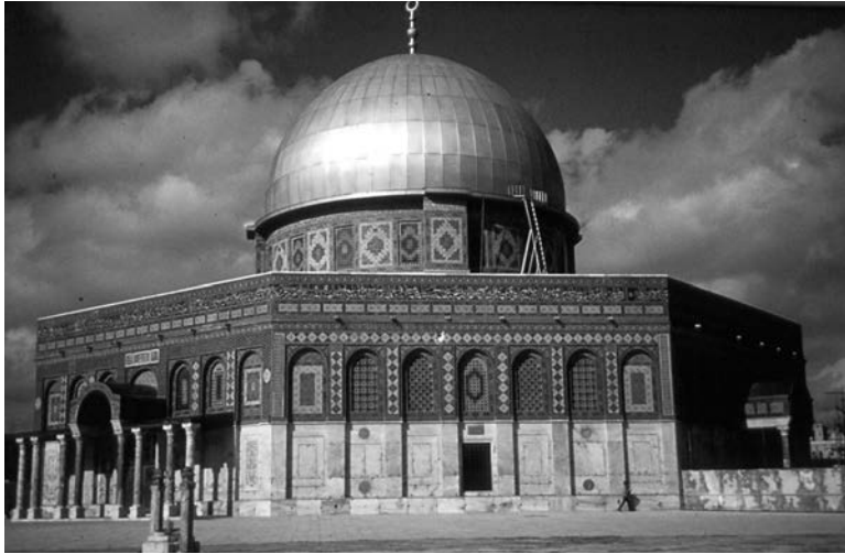
The Dome of the Rock in Jerusalem is considered to be the third most sacred site in Islam. It marks the site where Muhammad miraculously journeyed to heaven one night. The structure was restored during the Ottoman period. Photo: Kathleen Cohen.
